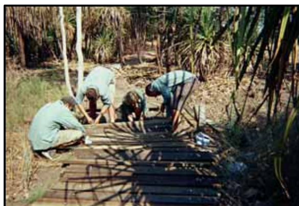
Green Corp members building the wooded walkway on Darwin International Airport land
