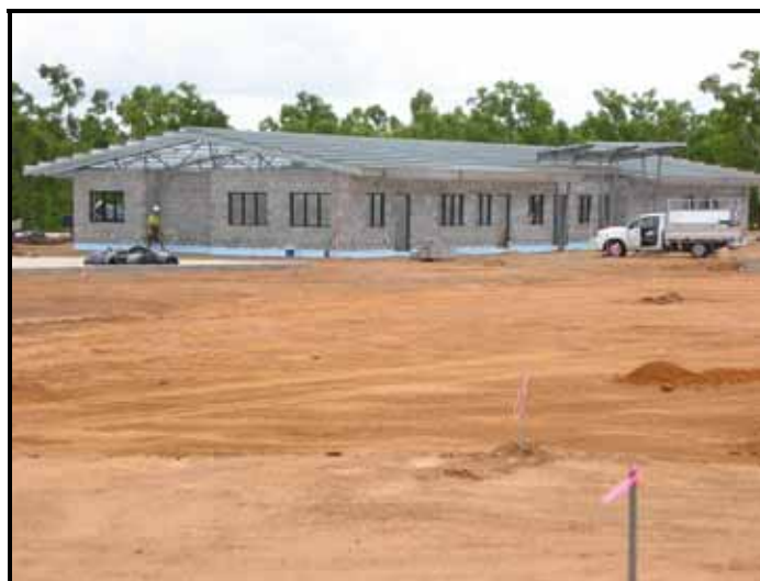
The Netball court complex under construction Rapid Creek is directly behind the complex, 27 November 2008
