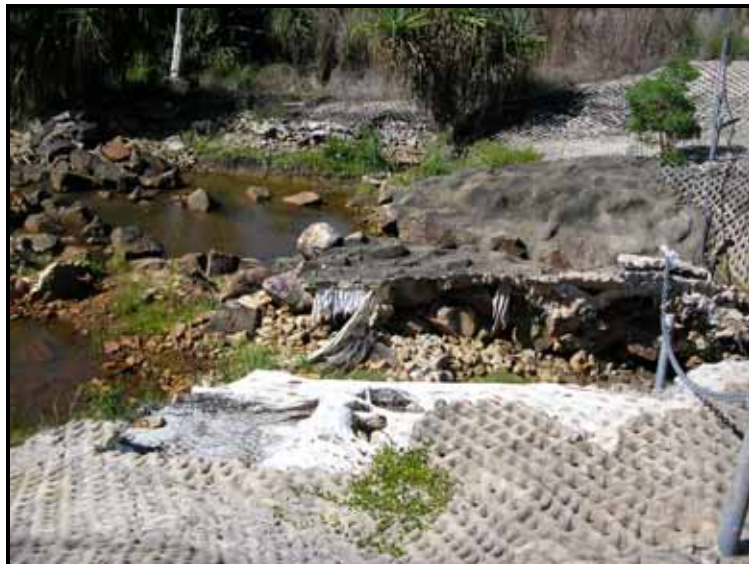
The damaged weir, 7 November 2008
