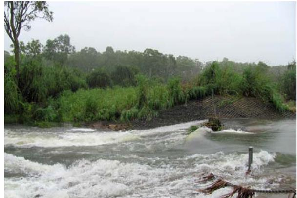
*Photos taken on the morning of Cyclone Carlos on 16/2/2011; the left photo shows the bank of the flood mitigation weir with debris demonstrating the water had come over the top; the right photo shows the creek channel coming through the weir (NB the flood peak had occurred the previous night)*
